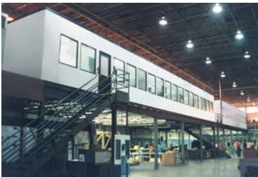
Offices on Pre-Engineered Mezzanine
