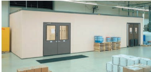
Vinyl finished ante room with painted steel doors and steel reinforced, impact doors.
