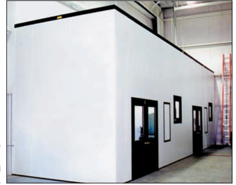
Negative pressure, HEPA filtered, Process Isolation Room with 3'x3' custom loading doors isolates grinding dust from plant ambient air.
