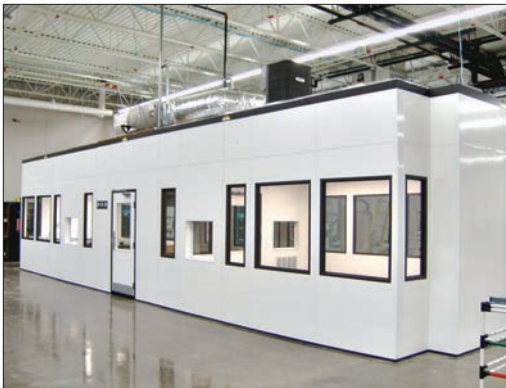
Cleanroom with internal ante room and dedicated HVAC system maintains Class 10,000 (ISO Class 7) conditions.
