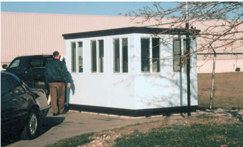
Visitor information building with many windows for borrowed light and visibility.
