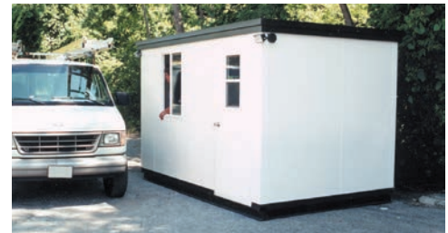
Security building with outdoor lighting.
